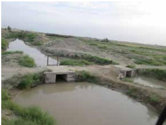
Figure 9: Distribution of water in Kang District. Unlike Zaranj, people do not have control gates for controlling amount of water, and they use such structures from clay or concret slabs for closing intakes.
