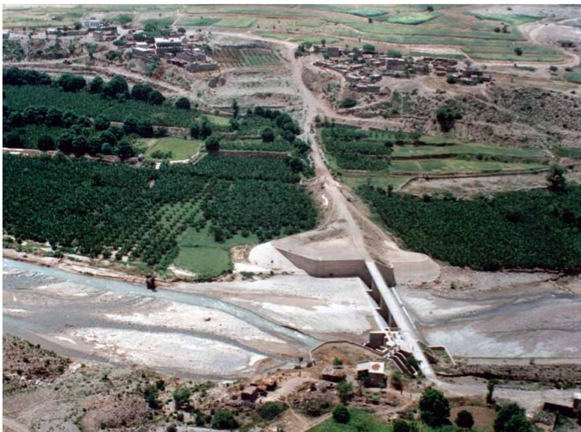
*Figure 5: Wadi Mawr Yemen: Weir blocking subsurface flows, benefitting upstream wells and land. Infrastructure development often undermine existing (informal) water rights and water distribution. It also often overlooks different elements of water control (f.i. subsurface flows) - creates voids and typically does not include work on modifying water rights and water distribution.*
