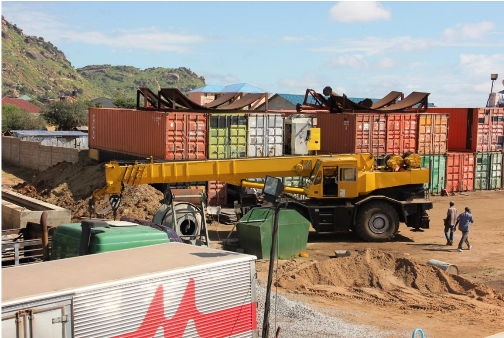
Photo 15: The construction yard of an upcoming local entrepreneur on the outskirts of Juba near the Jebel Kujur mountain.
